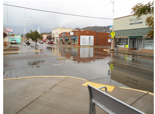
Ponding after a storm in Downtown.
